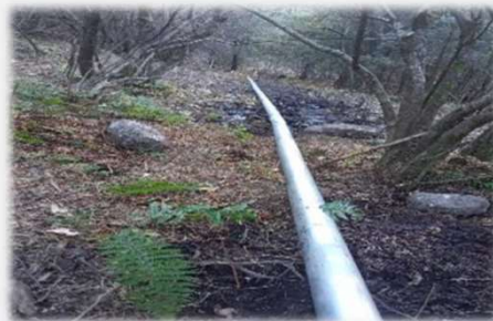
Laying of GMS Pipe
