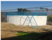
7 nos. of tanks with 4.5 Lakh Liters capacity has been constructed.
